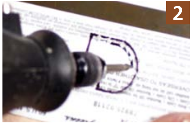
Cut out the opening, working inside the line.
